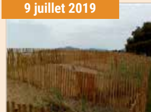
FIGURE 12: CHANGES TO THE SAND RIDGE FOLLOWING ON FROM THE REMOVAL OF RIPRAP AND THE ADDITION OF PICKET FENCES AT VIEUX-SALINS D'HYÈRES. © Conservatoire du littoral
